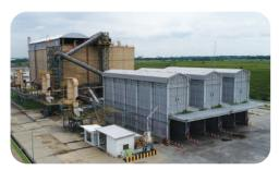
**Biomass Boiler technology**, by using rice husk as a fuel source to produce clean energy instead of using fuel oil
